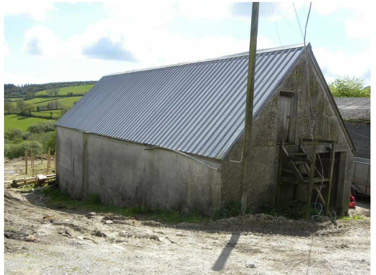
Box profile roof, concrete floor with electricity supply.
