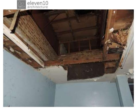
Damaged ceilings to the existing first floor and exposed second floor above
