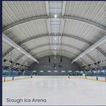
Slough Ice Arena
