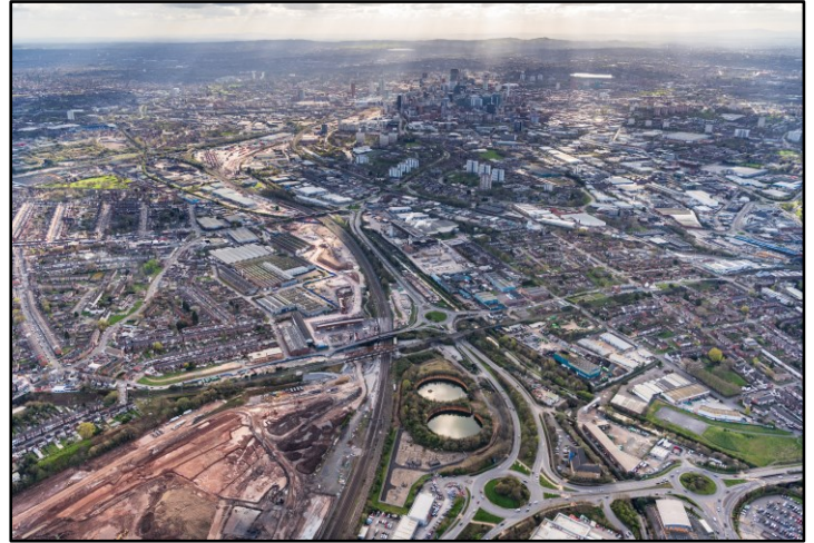
View of the Site from the East
