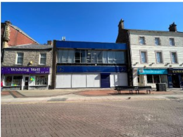
Front elevation on Bedford Street
