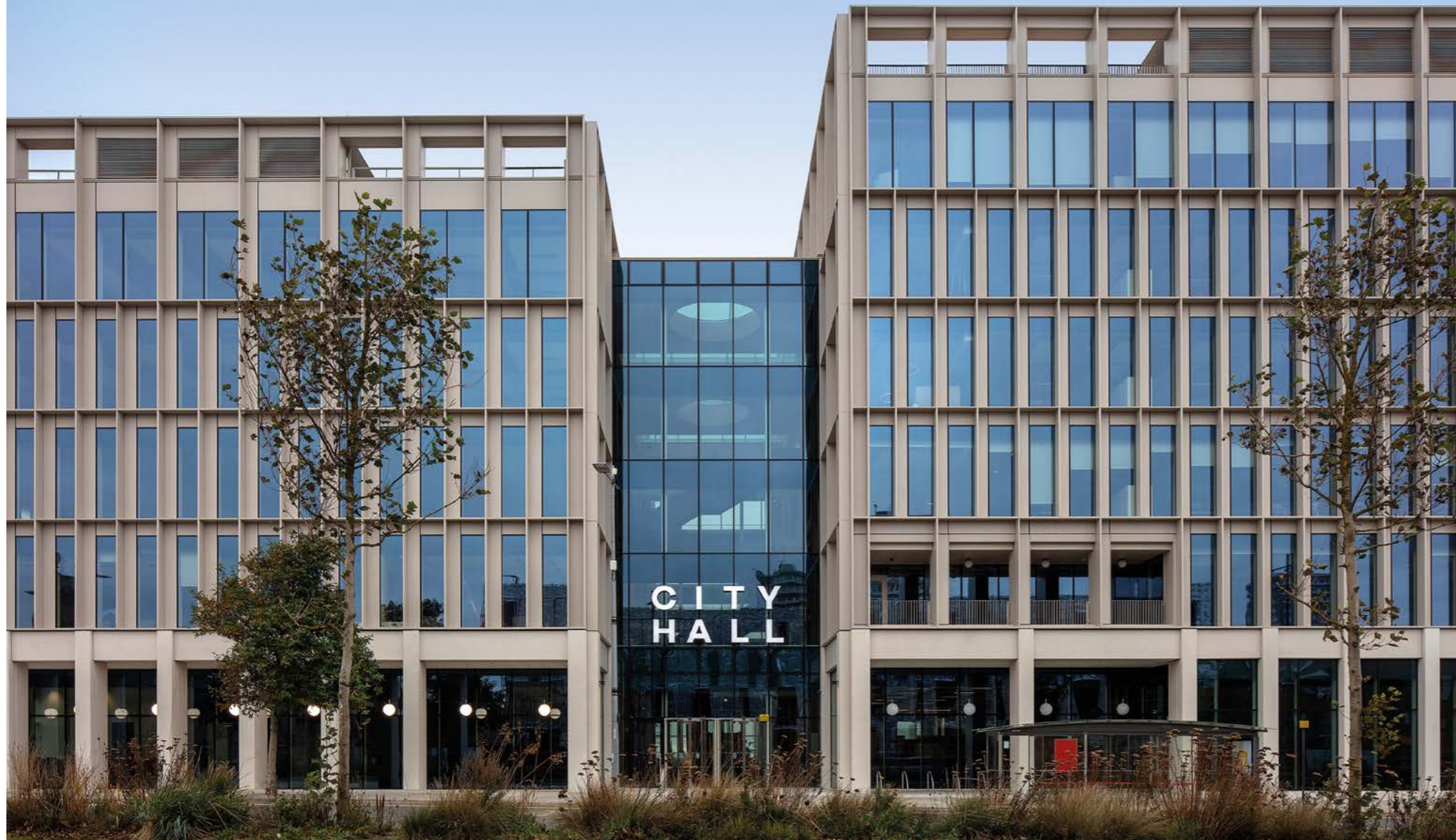
1. The City Hall building
