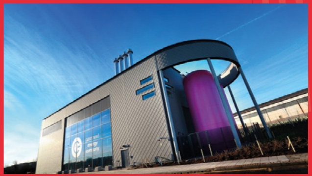
District Energy Centre
