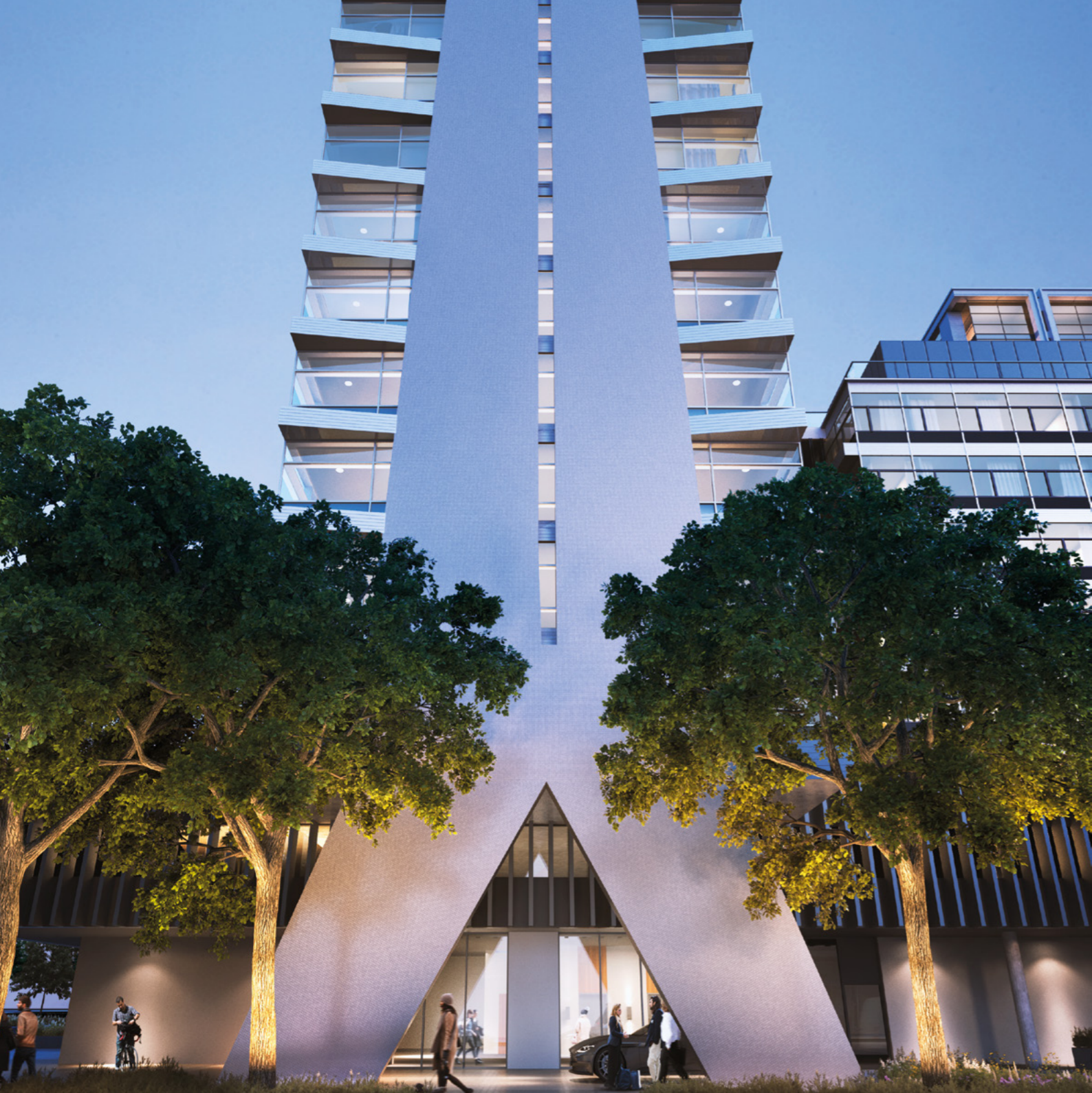
Left A modern makeover for a modernist icon; the inimitable architecture of Tolworth Tower.
