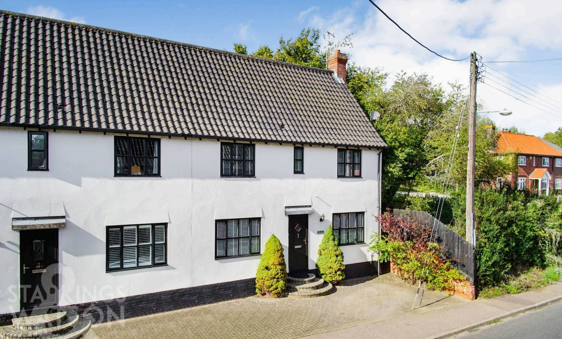
The Street, Brockdish - IP21 4JY
