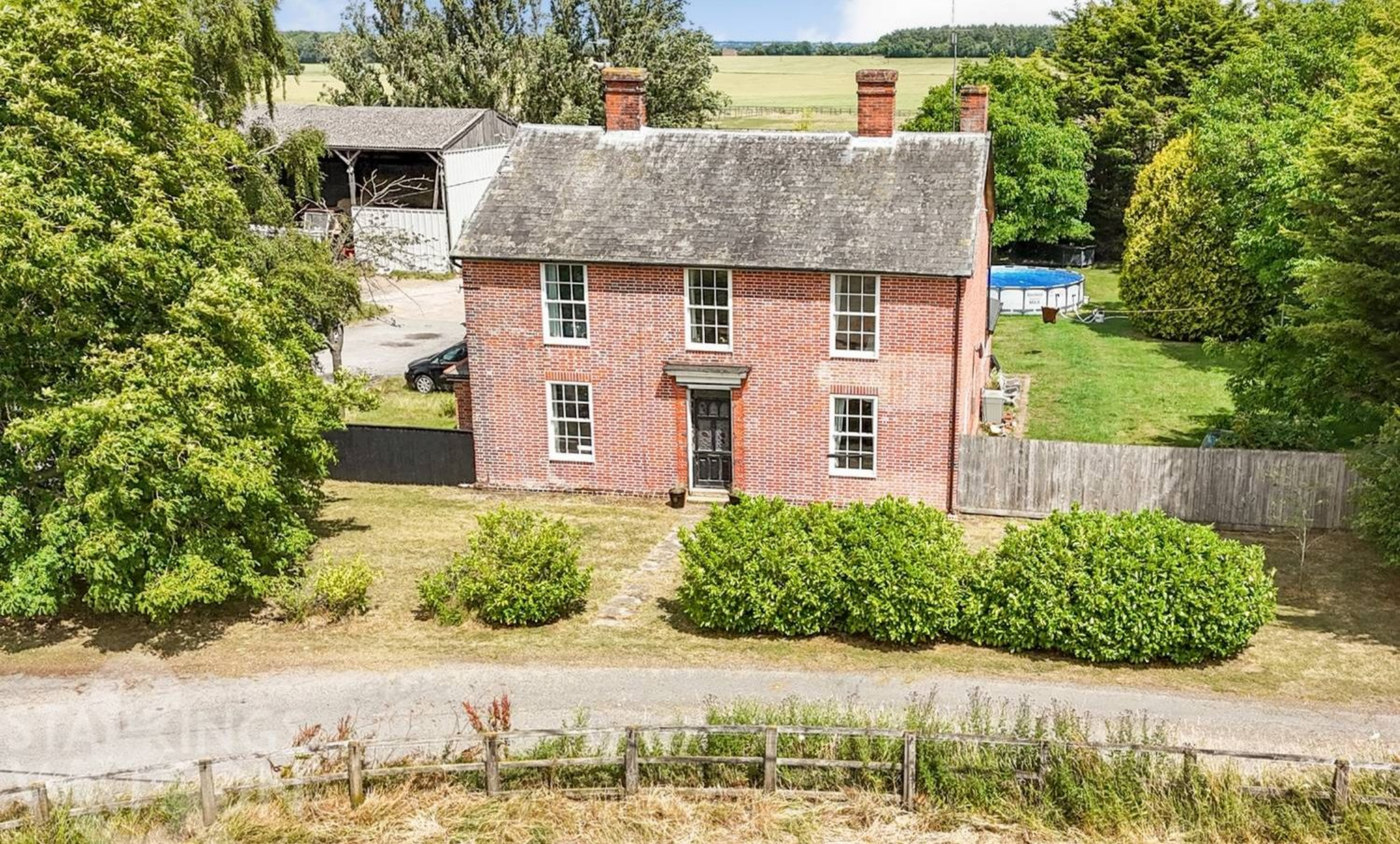
Church Lane, Hepworth - IP22 2QE
