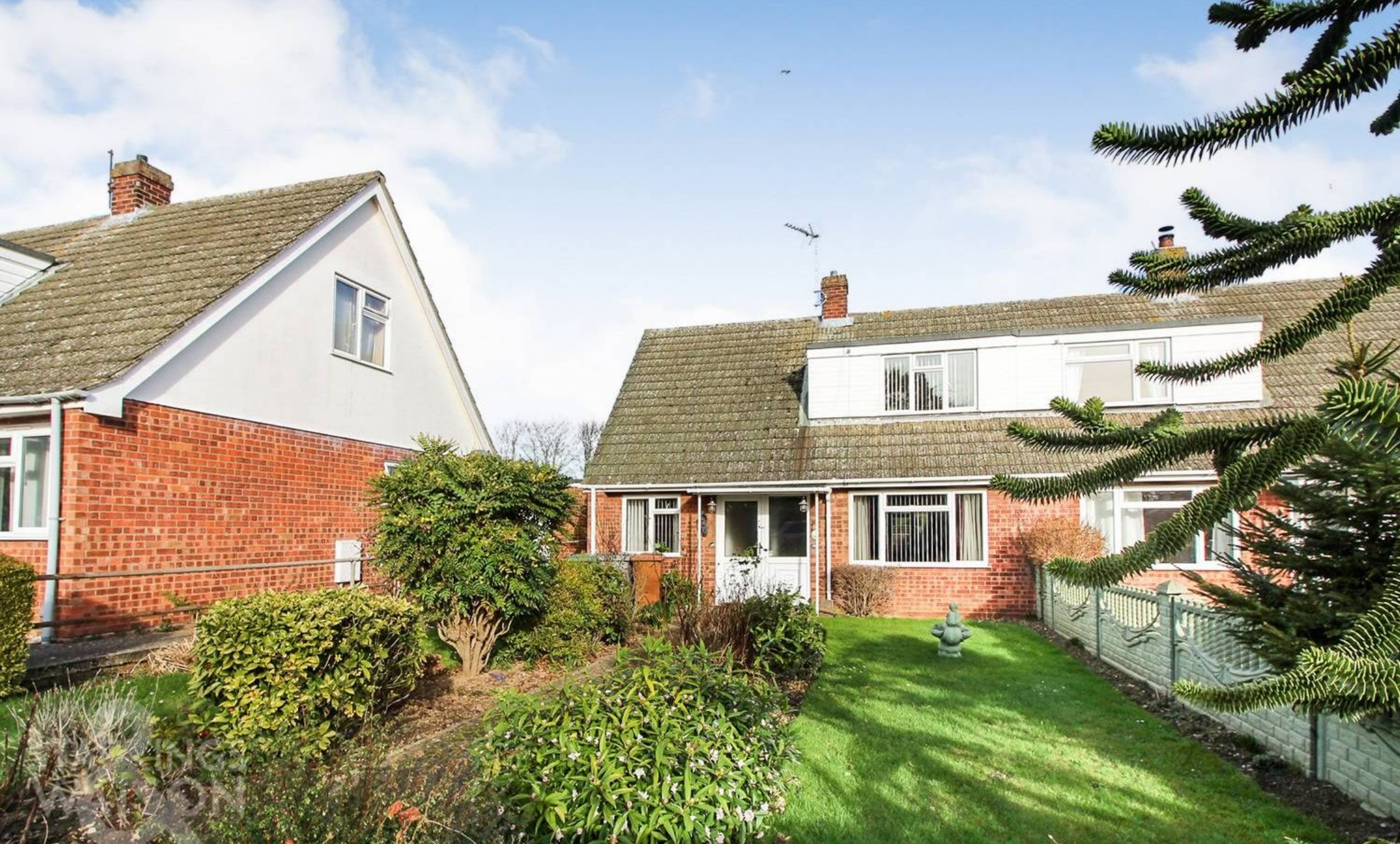
Springdale Crescent, Brundall - NR13 5RA
