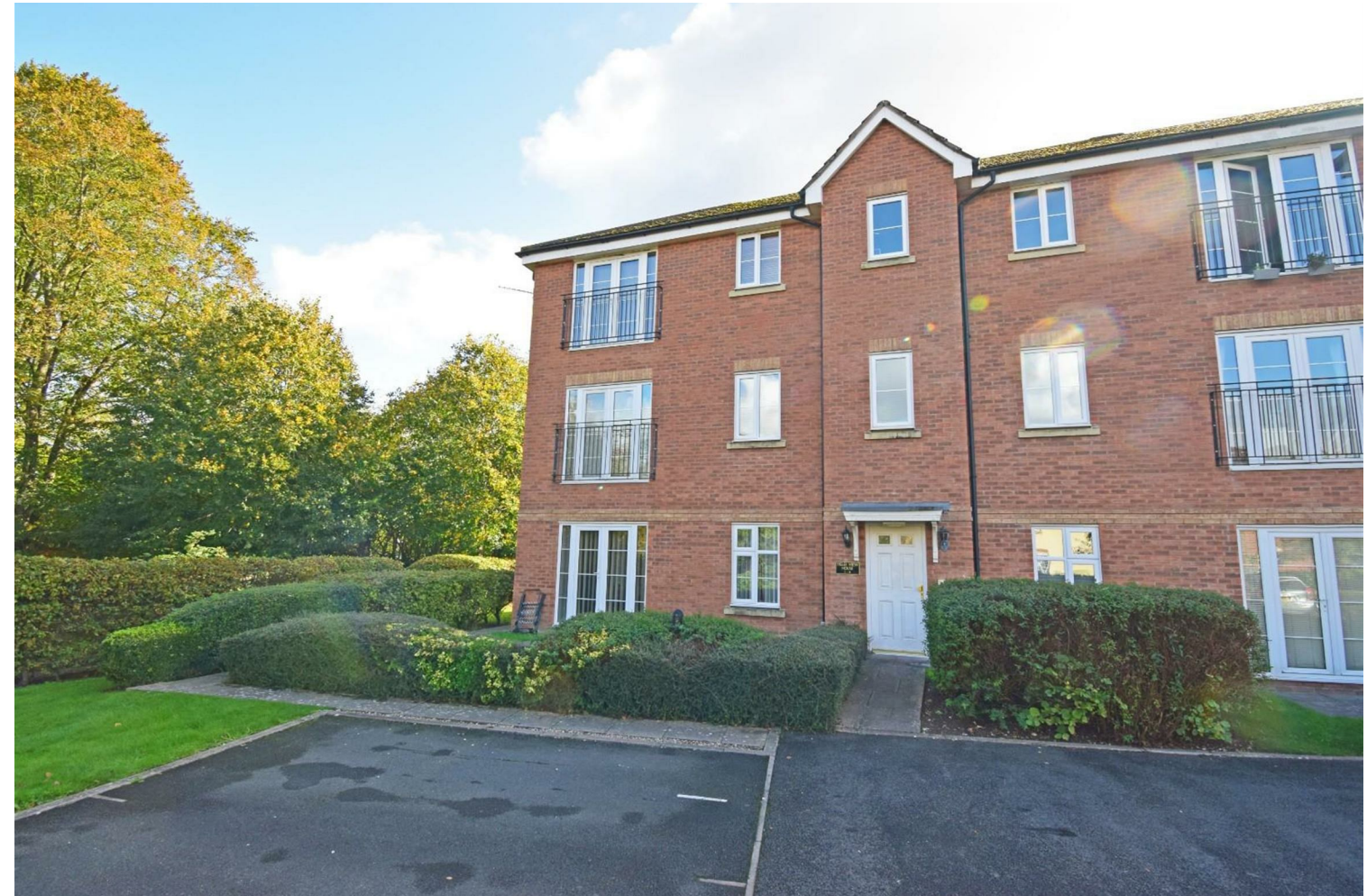
1 Field View House, Railway Walk, Bromsgrove, B60 3GY
