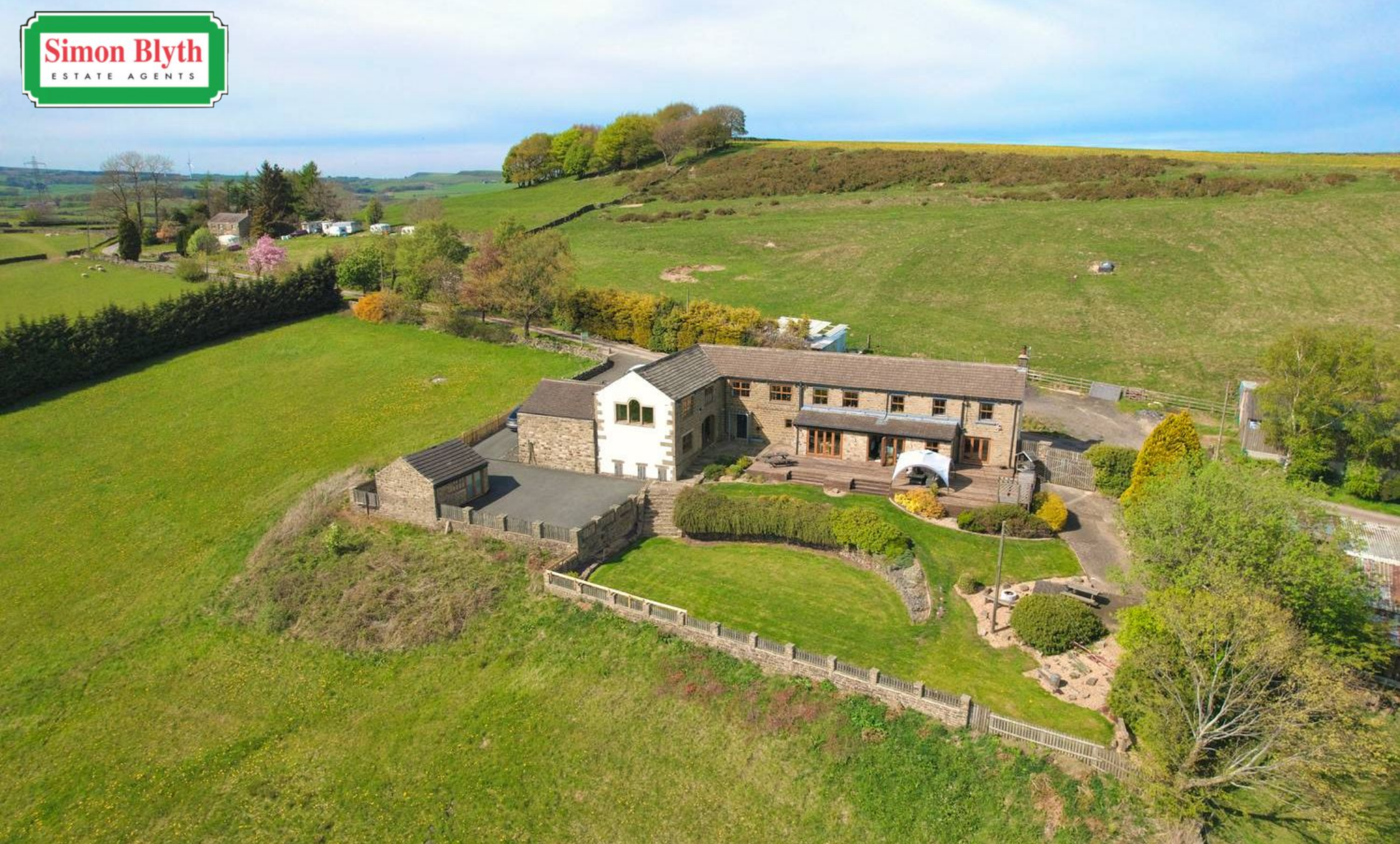
Cote Farm, Nether House Lane Sheffield
