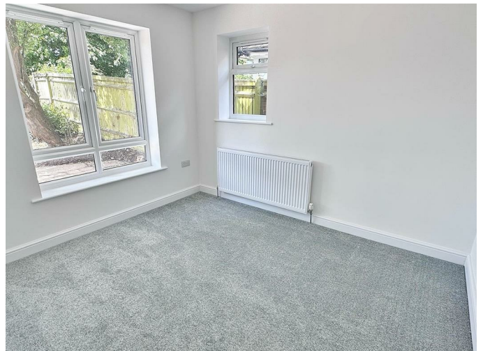
Radiator. uPVC double glazed windows to front and side.
