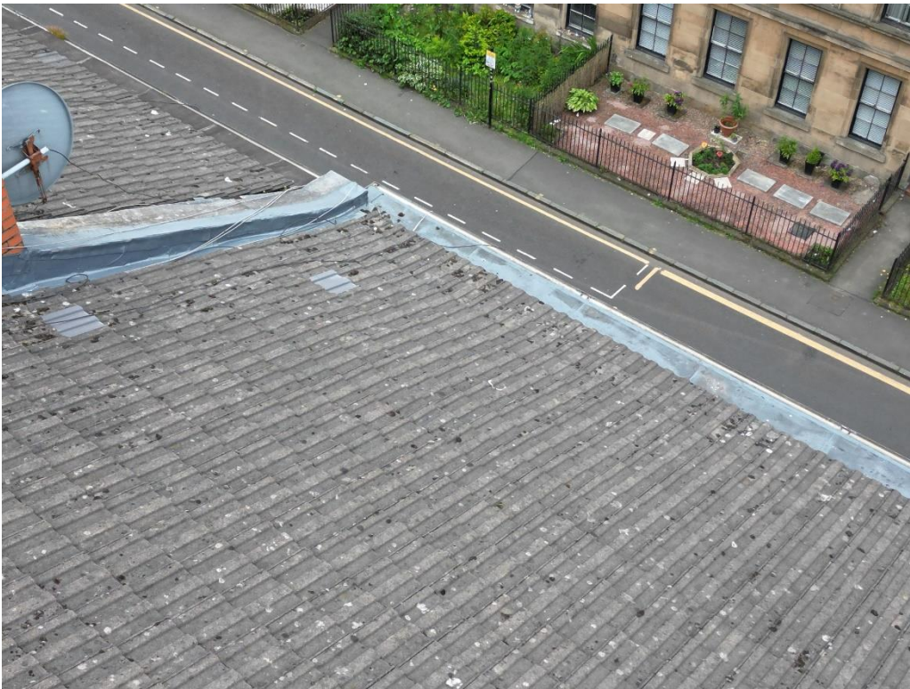
Dilapidated front lead deck
