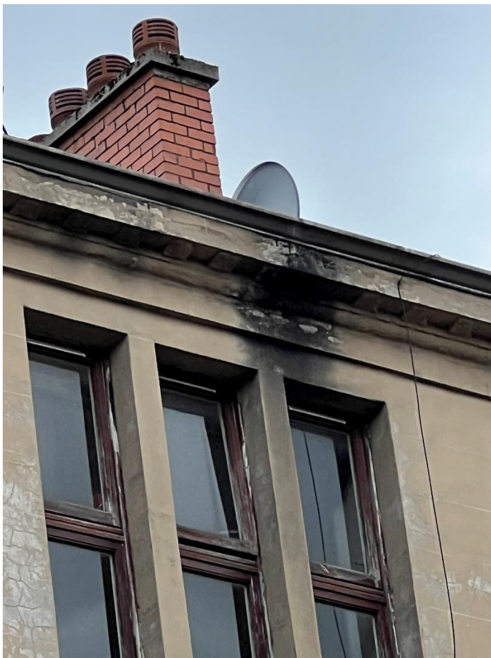
Example of leaking guttering with no undercloak
