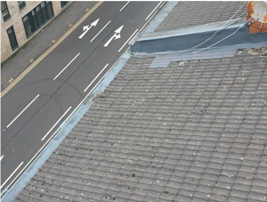
“Painted” parapet gutter deck and skew
