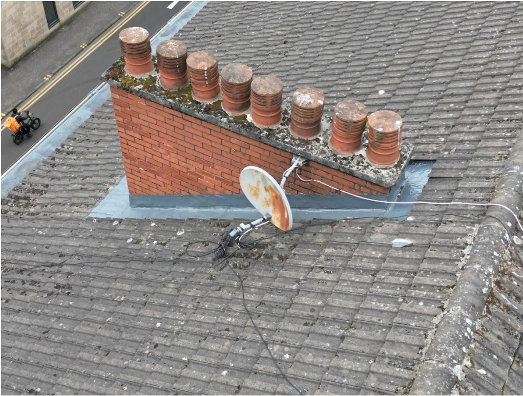
“Painted” chimneyhead flashing
