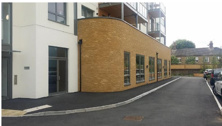
Entrance to Dairy Court 2 car spaces available
