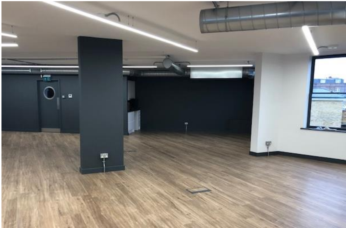
Third Floor with floor boxes
