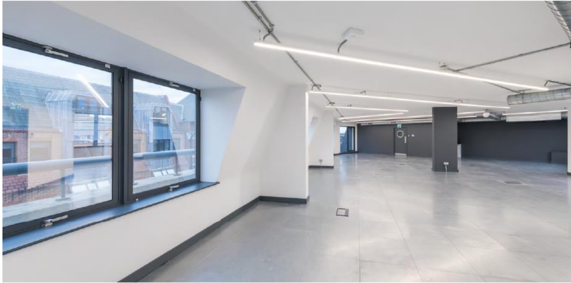
Third floor before laminate floor
