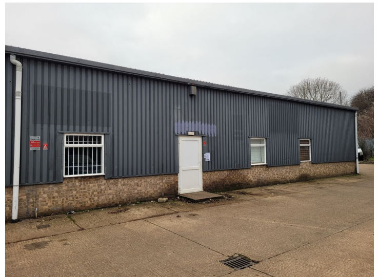
Photo above shows Unit 11.
