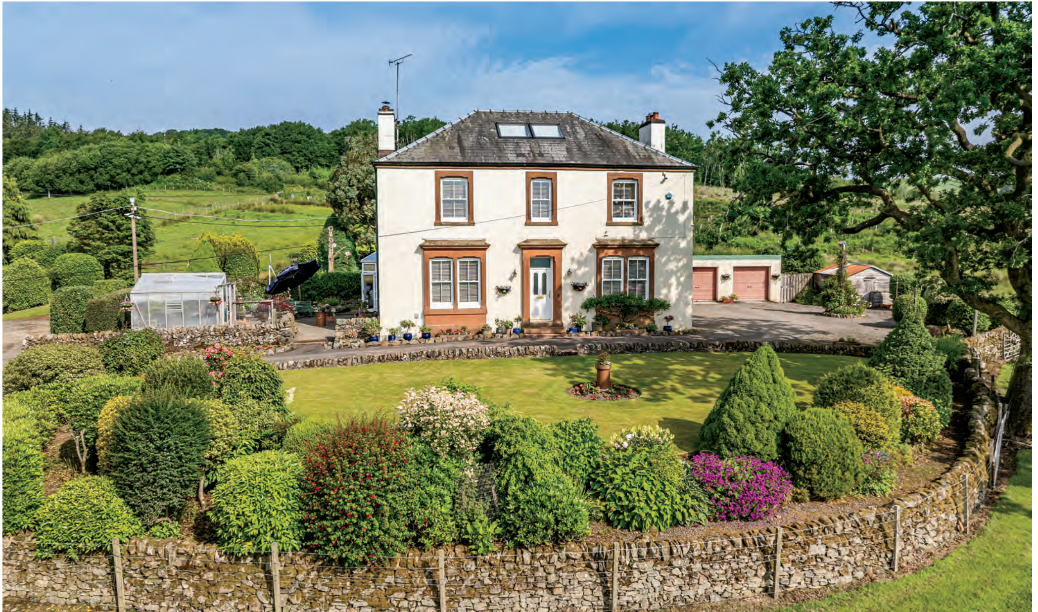
Larglanglee House Crocketford | Dumfries | DG2 9ST
