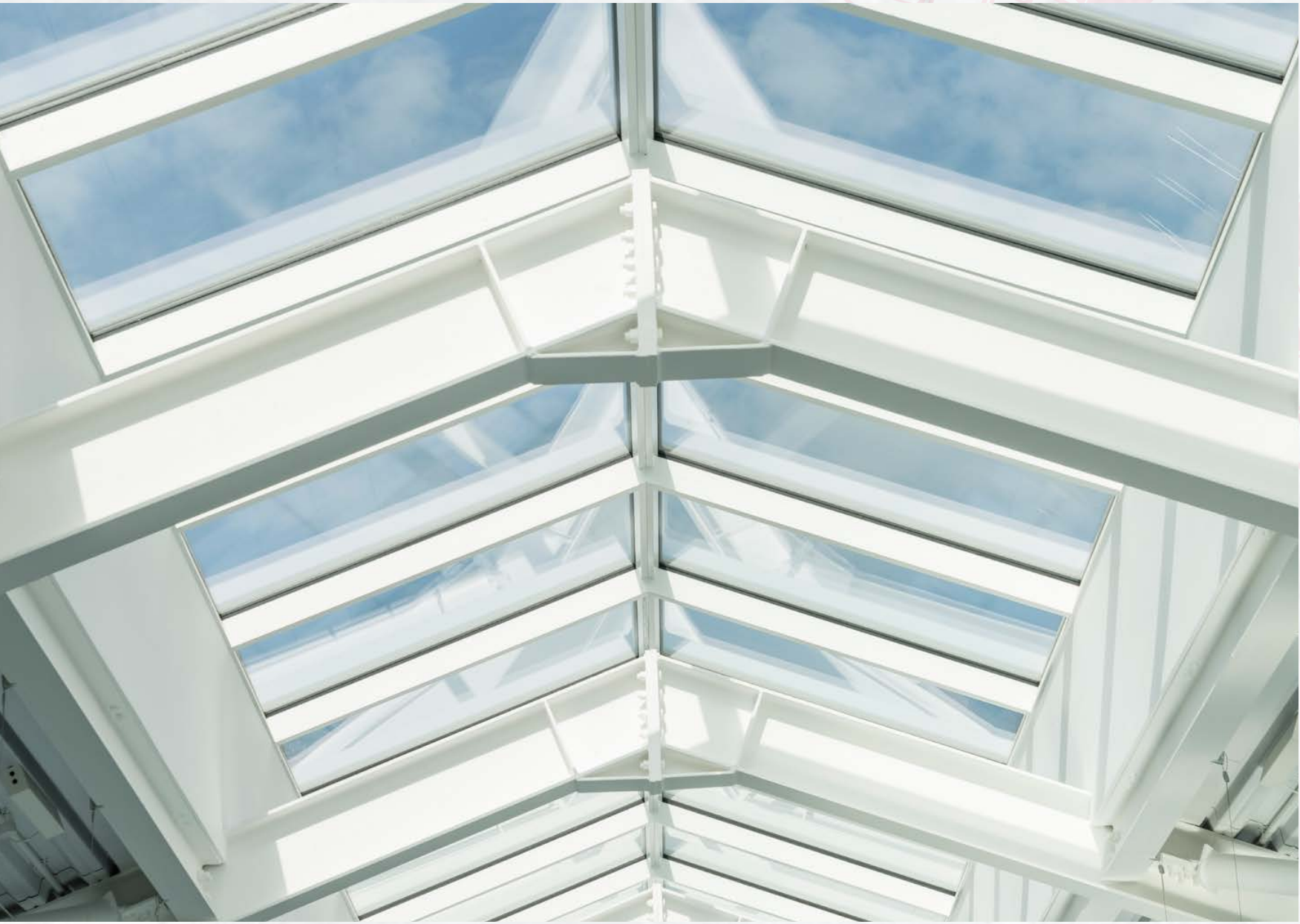
Second floor skylight
