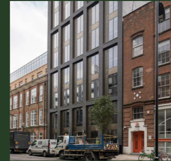
6th floor Verse Building, N1
