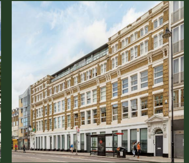
1st floor 78 Kingsland Road, E2
