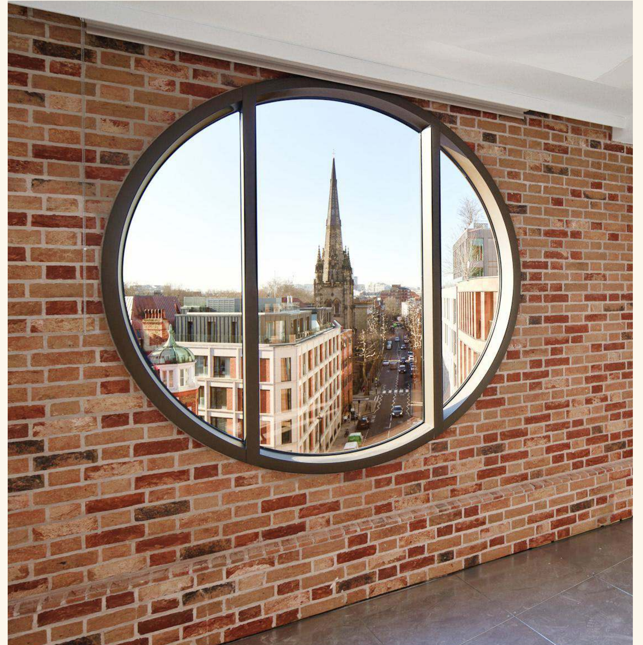
Fifth Floor windows
