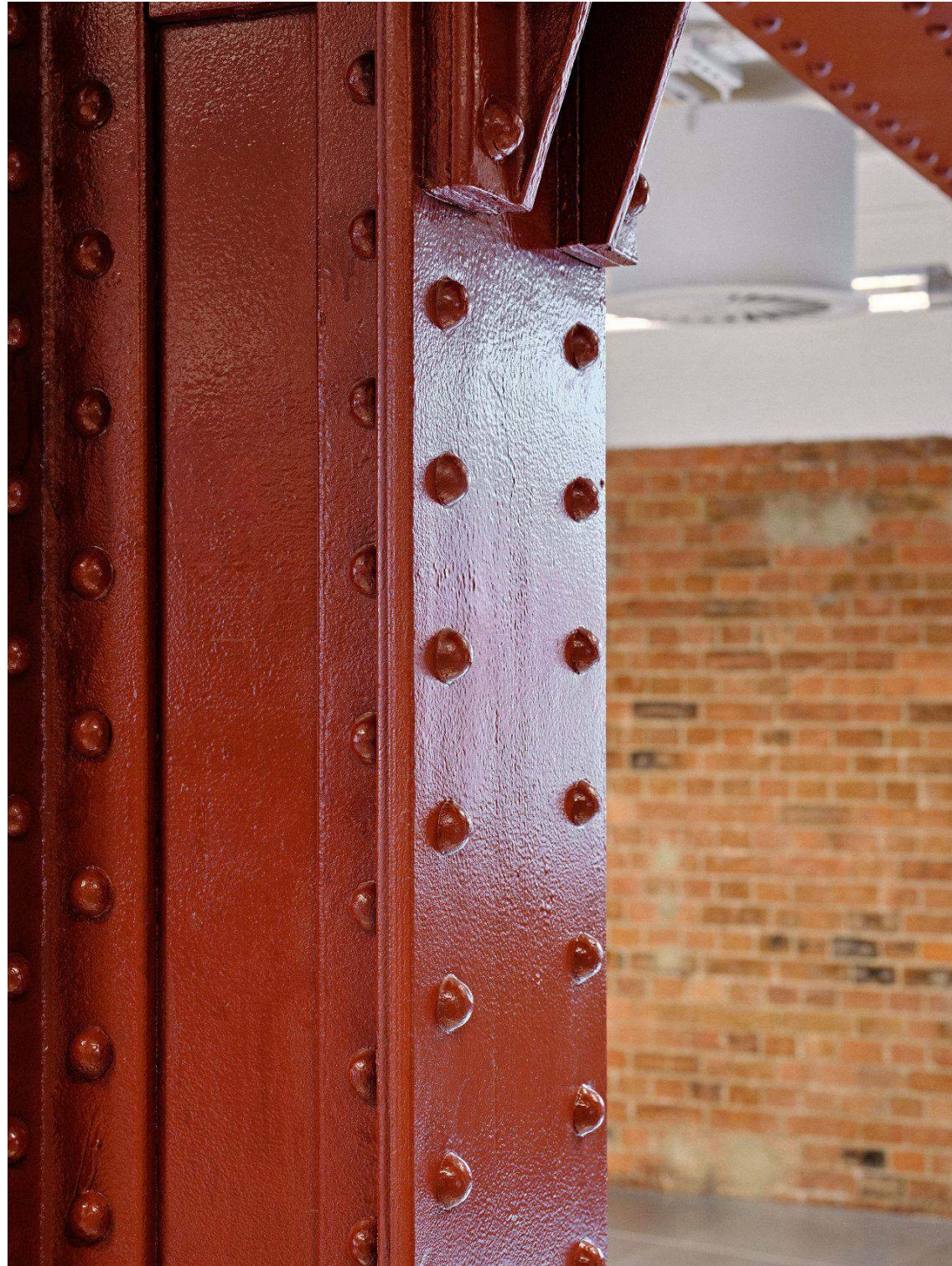
Retained steel columns
