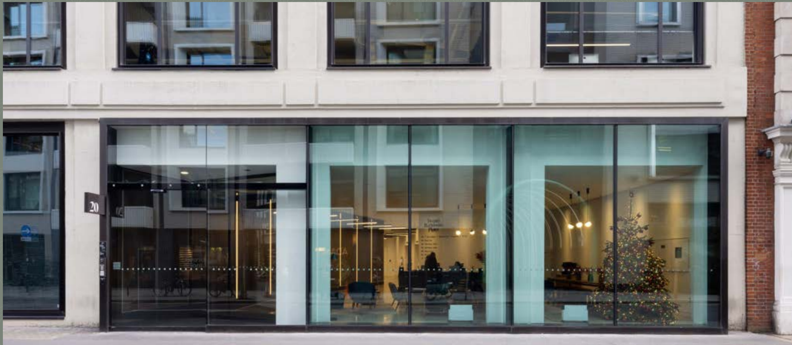
GROUND FLOOR FAÇADE
