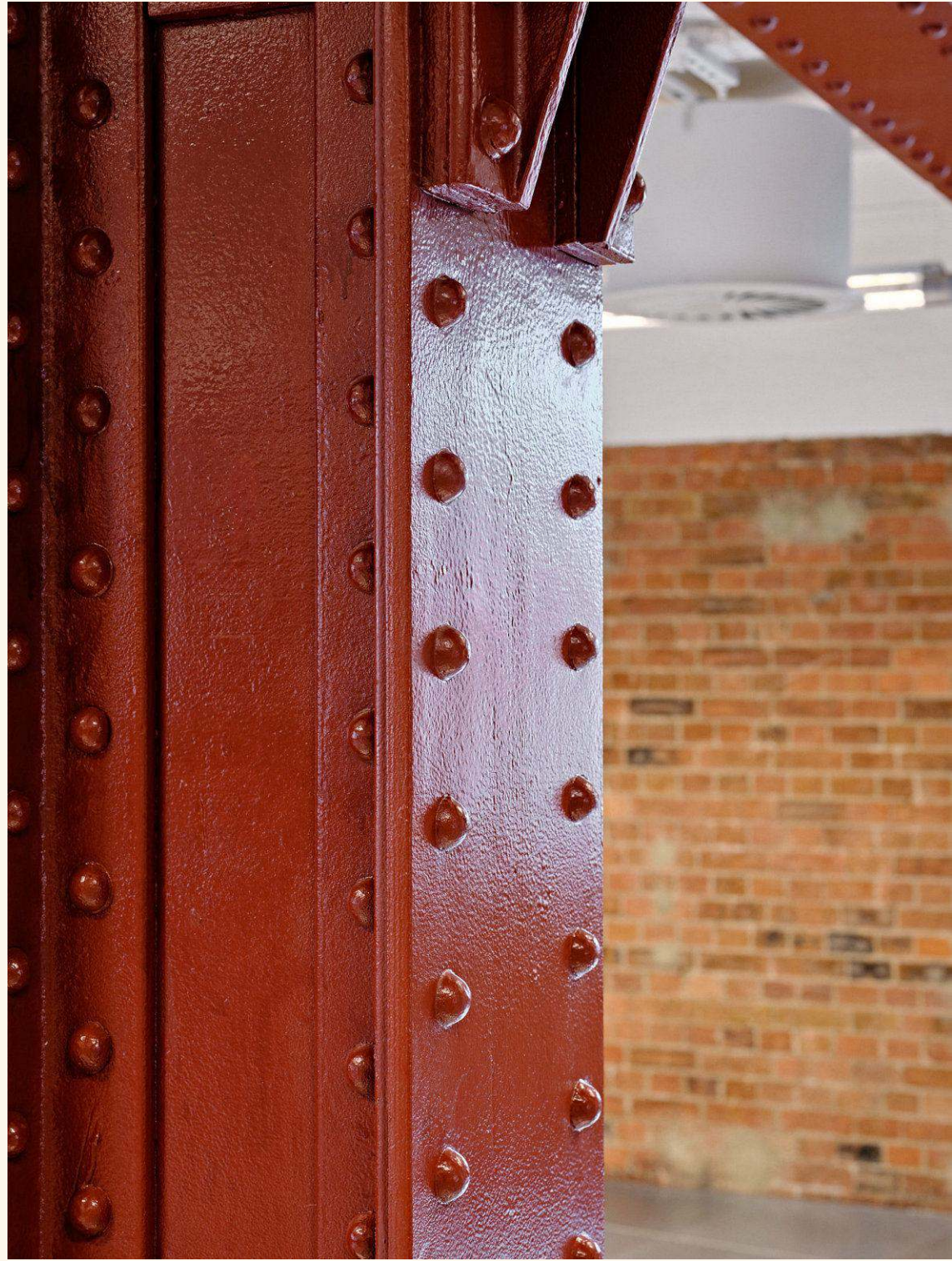
Retained steel columns
