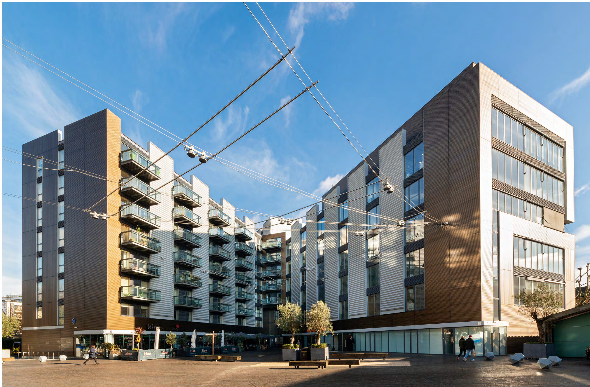
View across Bermondsey Square, to the offices
