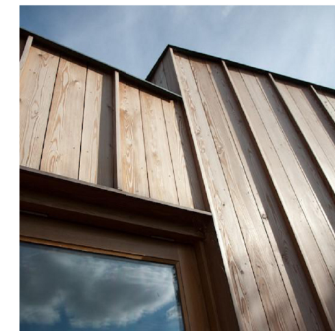
Board and batten larch cladding - references tudor style timber panellings
