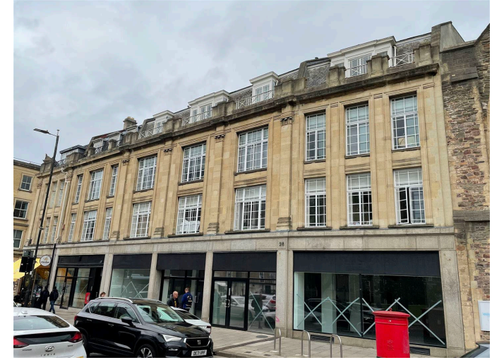
Unit 1 and 2 & Basement
