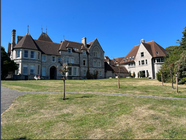
Rear View of Main House and Extension
