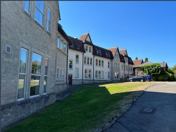
External View of Extension and Stables
