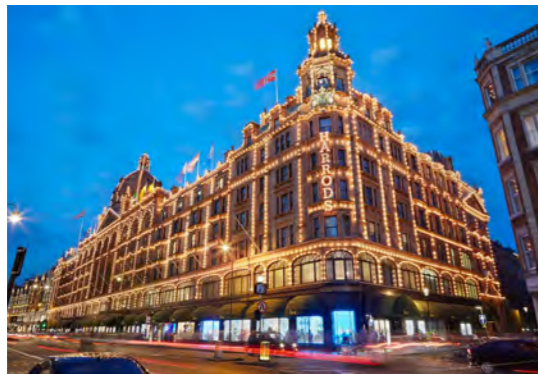
Harrods Department store
