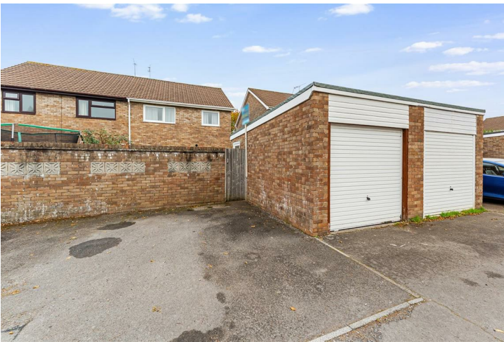
Garage located at the rear of the property being single in length. Accessed via an up and over door with light and power connected and window and pedestrian door. There is adjacent parking.
