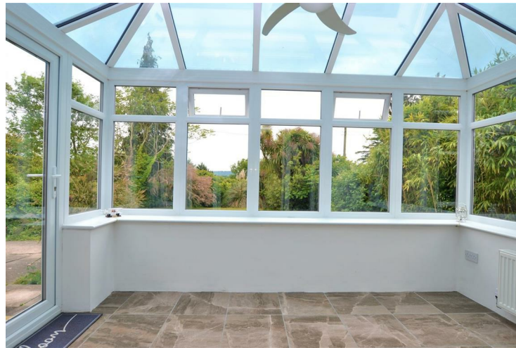
Of UPVC double glazed construction with dwarf walls and glass roof. Radiator, ceiling fan, tiled flooring and UPVC double glazed door to the front.
