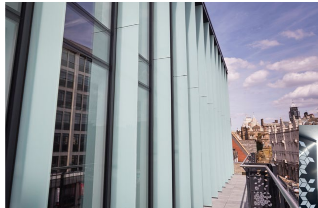
Upper balcony with views over Greek Street and East Parade
