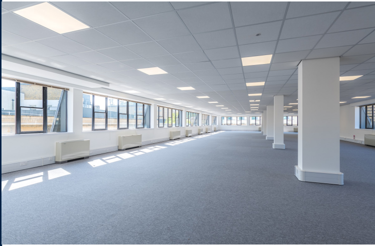
3rd Floor refurbishment (Jan 2024)
