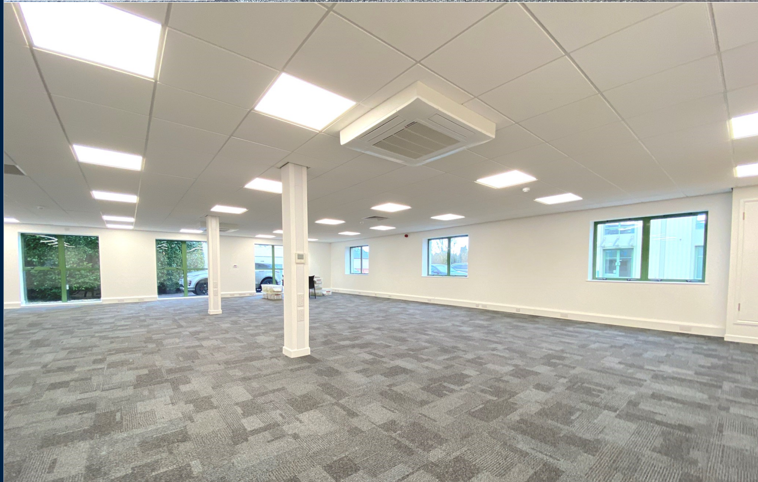
Unit 7 - Ground floor refurbishment
