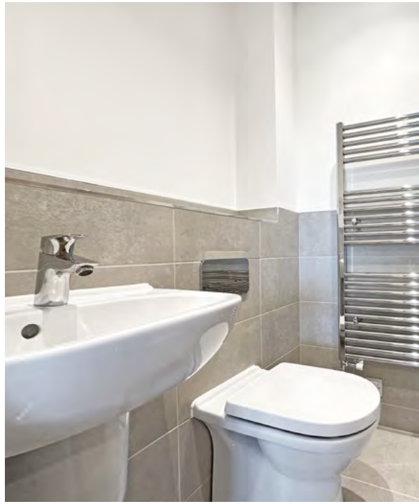
Modern White Villeroy and Boch sanitaryware
