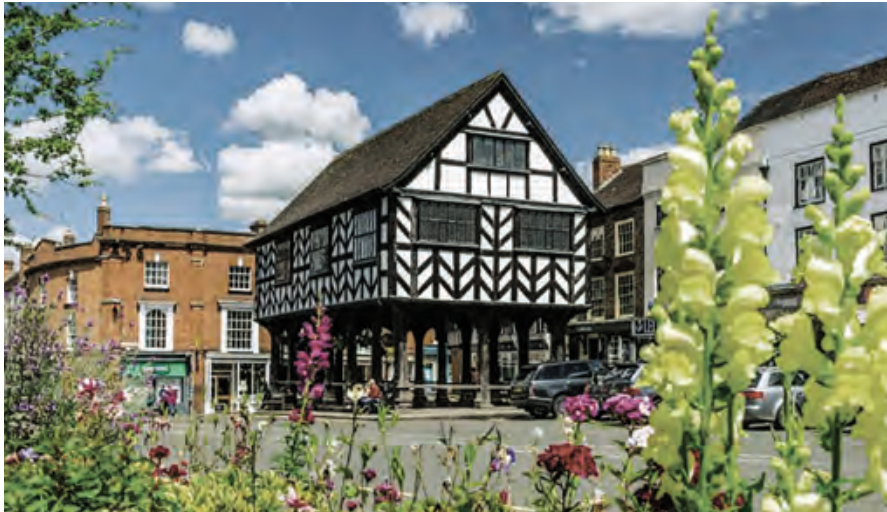
Ledbury 17C Market House
