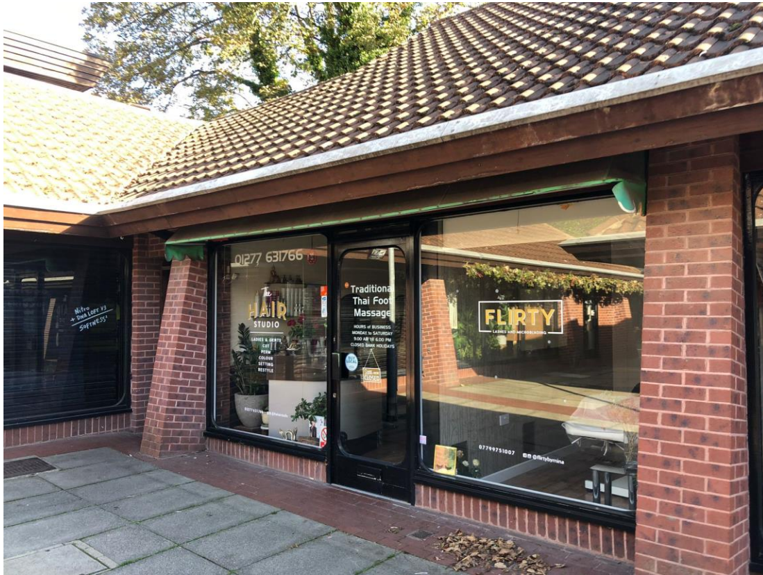
Unit 7 The Walk: Hair Salon Ground Floor: 44 sq m (474 sq ft) Open plan retail, Storage, Kitchenette
