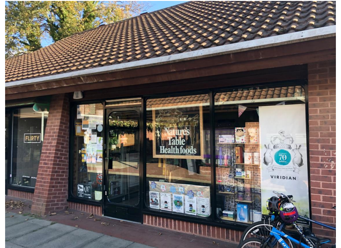
Unit 8 The Walk: Organic Food Supplements Ground Floor: 45 sq m (485 sq ft) Open plan retail, Storage, Kitchenette
