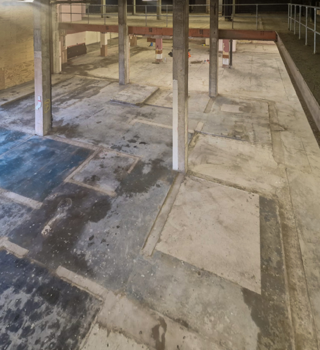
Former Bingo Hall, Chelmsley Wood Shopping Centre, Birmingham B37 5TT
