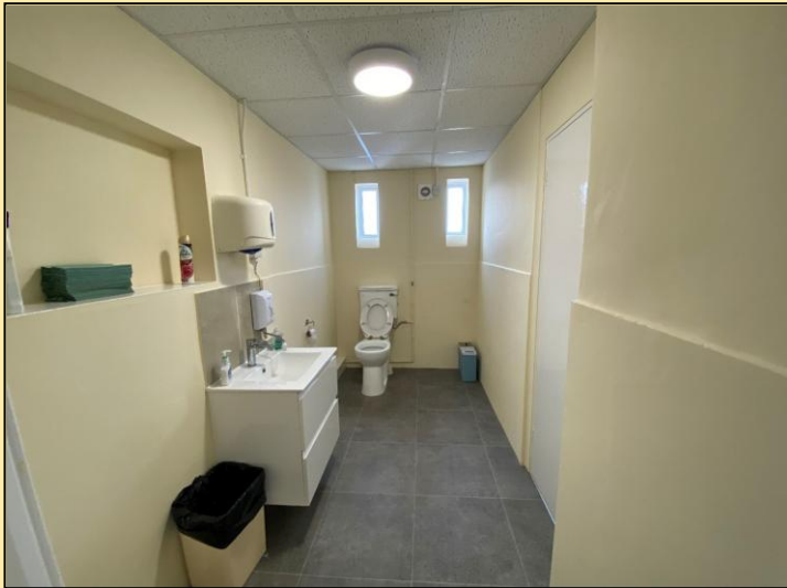
GROUND FLOOR WASHROOM
