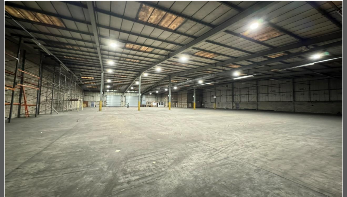
Image taken prior to refurbishment
