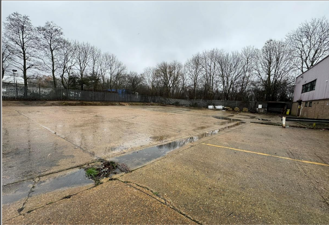
Image taken prior to refurbishment
