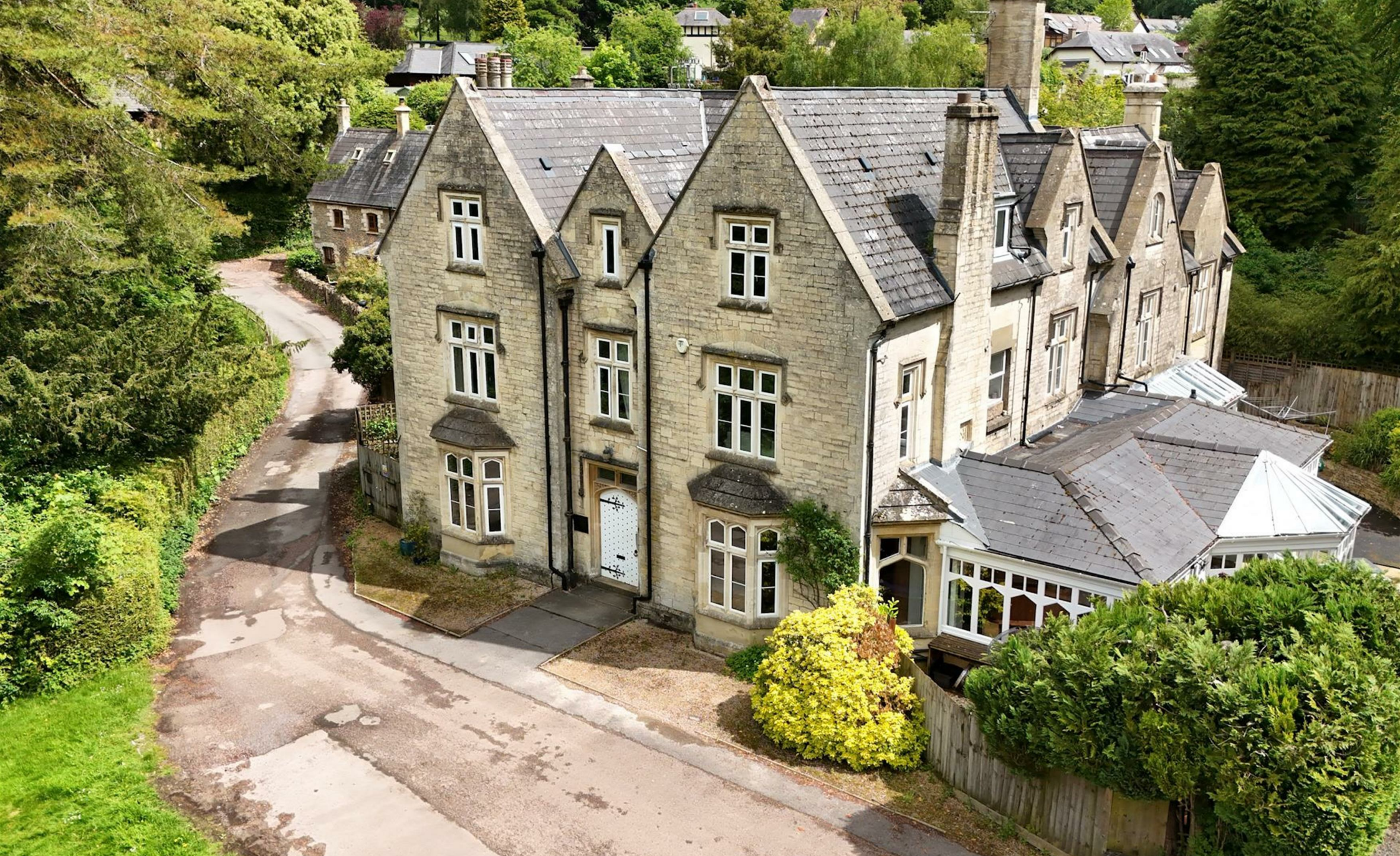
Flat 4 Salterley Grange Apartments, Leckhampton Hill, Cheltenham, GL53 9QW
