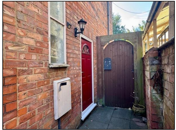
SIDE ENTRANCE DOOR
