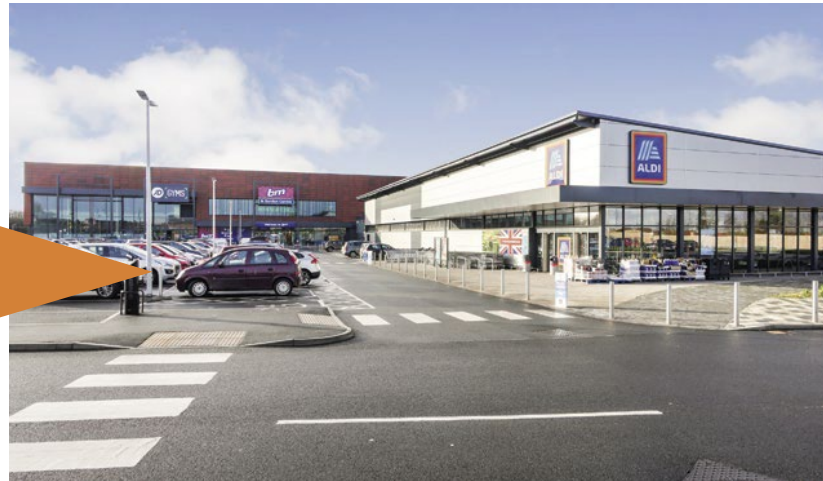
Northumberland Retail Park - 50,000 sq ft retail/leisure development due for completion September 2019. The scheme will complement the existing 19,000 sq ft Aldi, Costa drive-thru and 21,368 sq ft retail parade anchored by a 24,772 sq ft Sainsbury's Store
