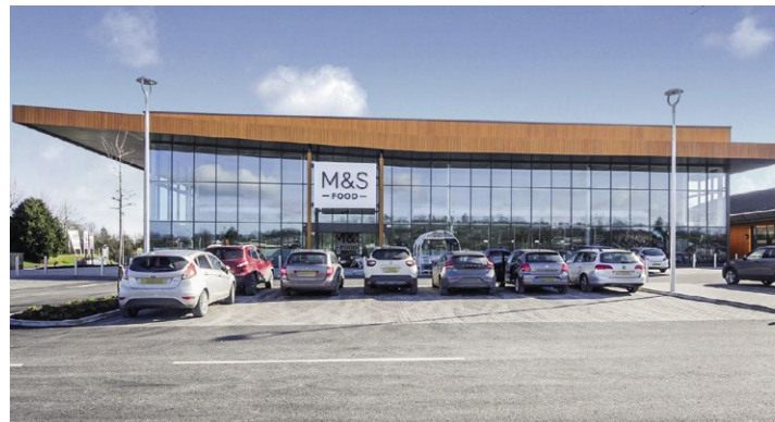
Willowburn Retail Park - Phase 1 due for completion August 2019 to provide 12,000 sq ft M&S Food Hall, Starbucks drive-thru and local artisan country store. Phase 2 will deliver an additional 20,000 sq ft of retail premises
