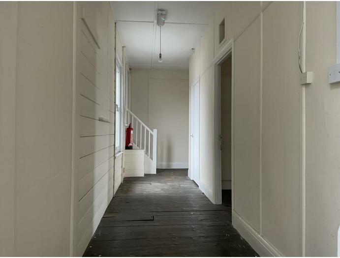
Doors to (right to left)
