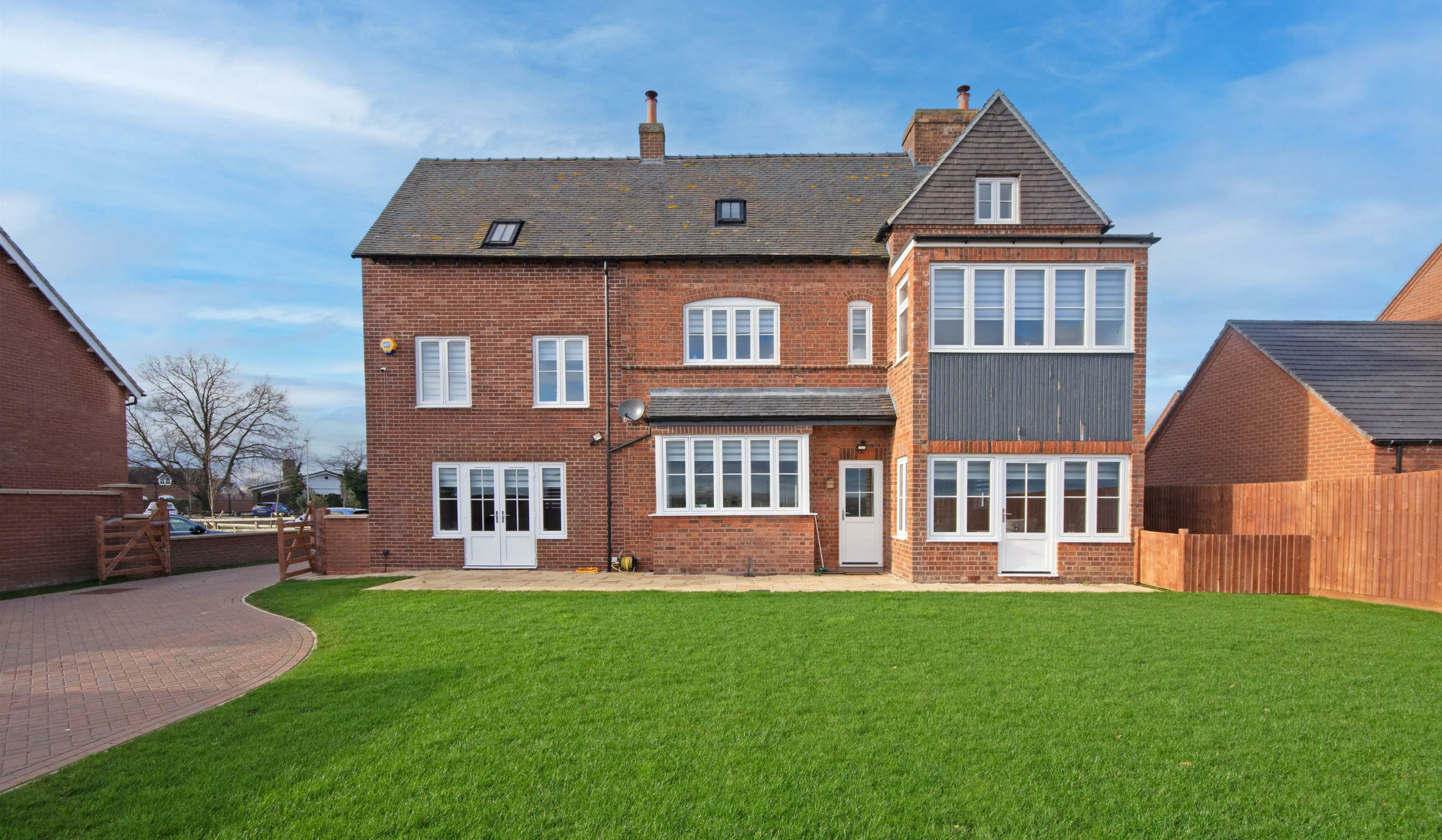
HIGHFIELD HOUSE, MANOR LANE HARLASTON, TAMWORTH
