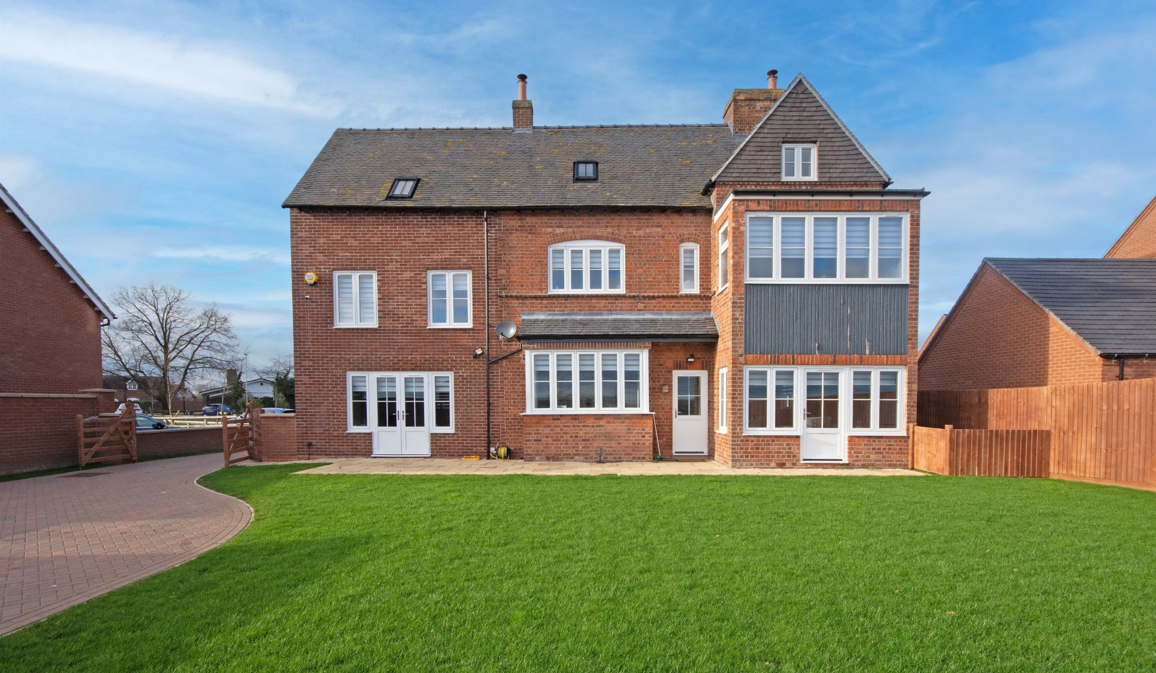
HIGHFIELD HOUSE, MANOR LANE HARLASTON, TAMWORTH
