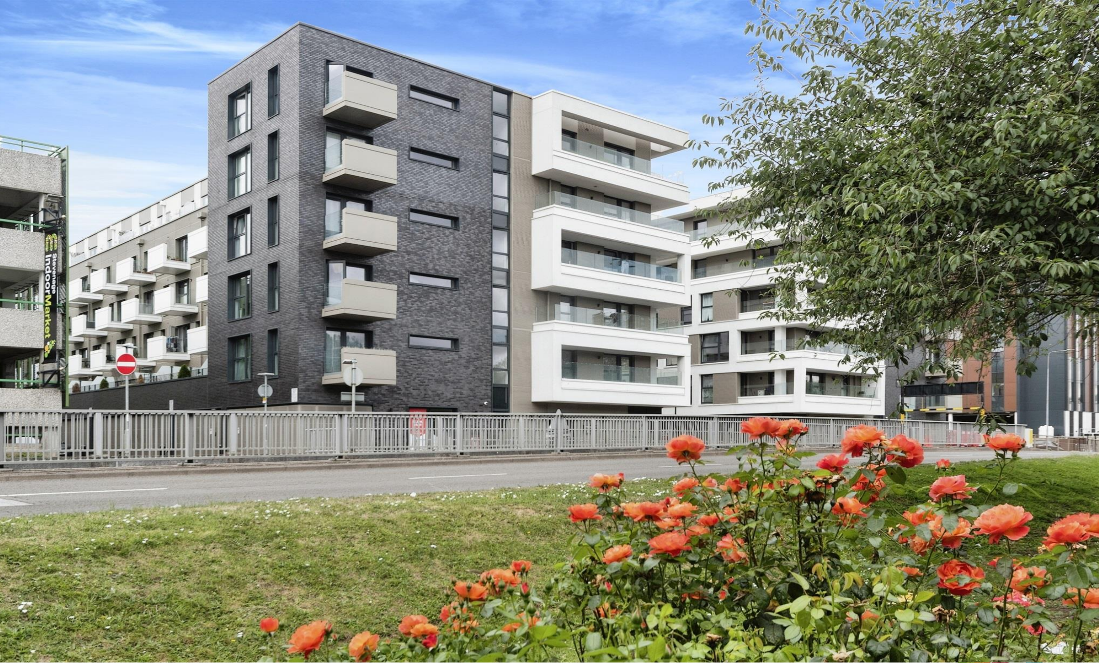
Mulberry House, Park Place, Stevenage SG1 1BH
