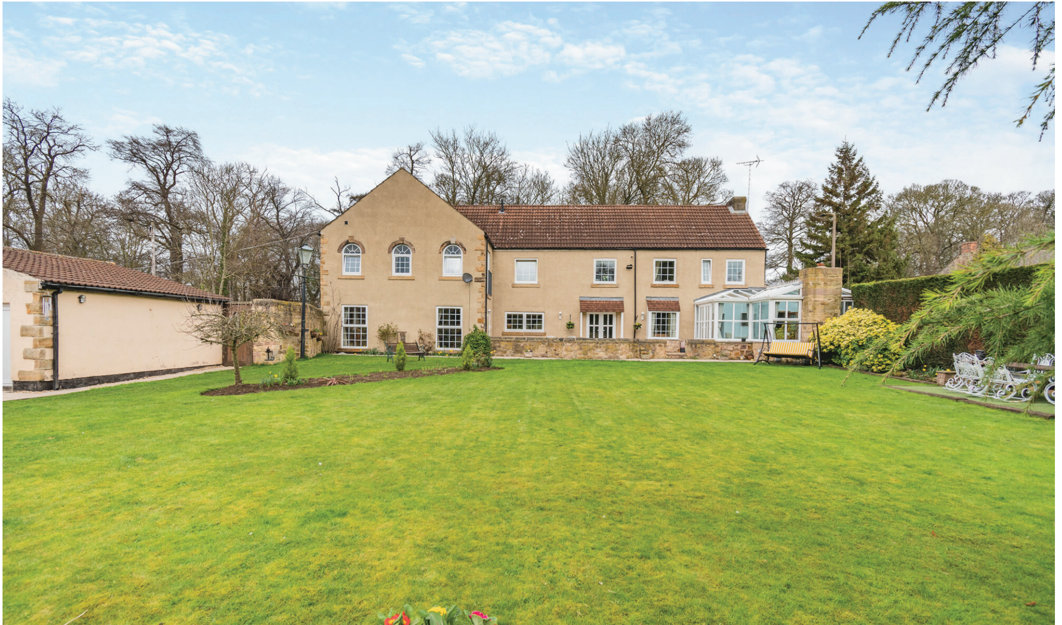
Beck View Cottage 1 Kilnhurst Road | Hooton Roberts | Rotherham | S65 4PE
