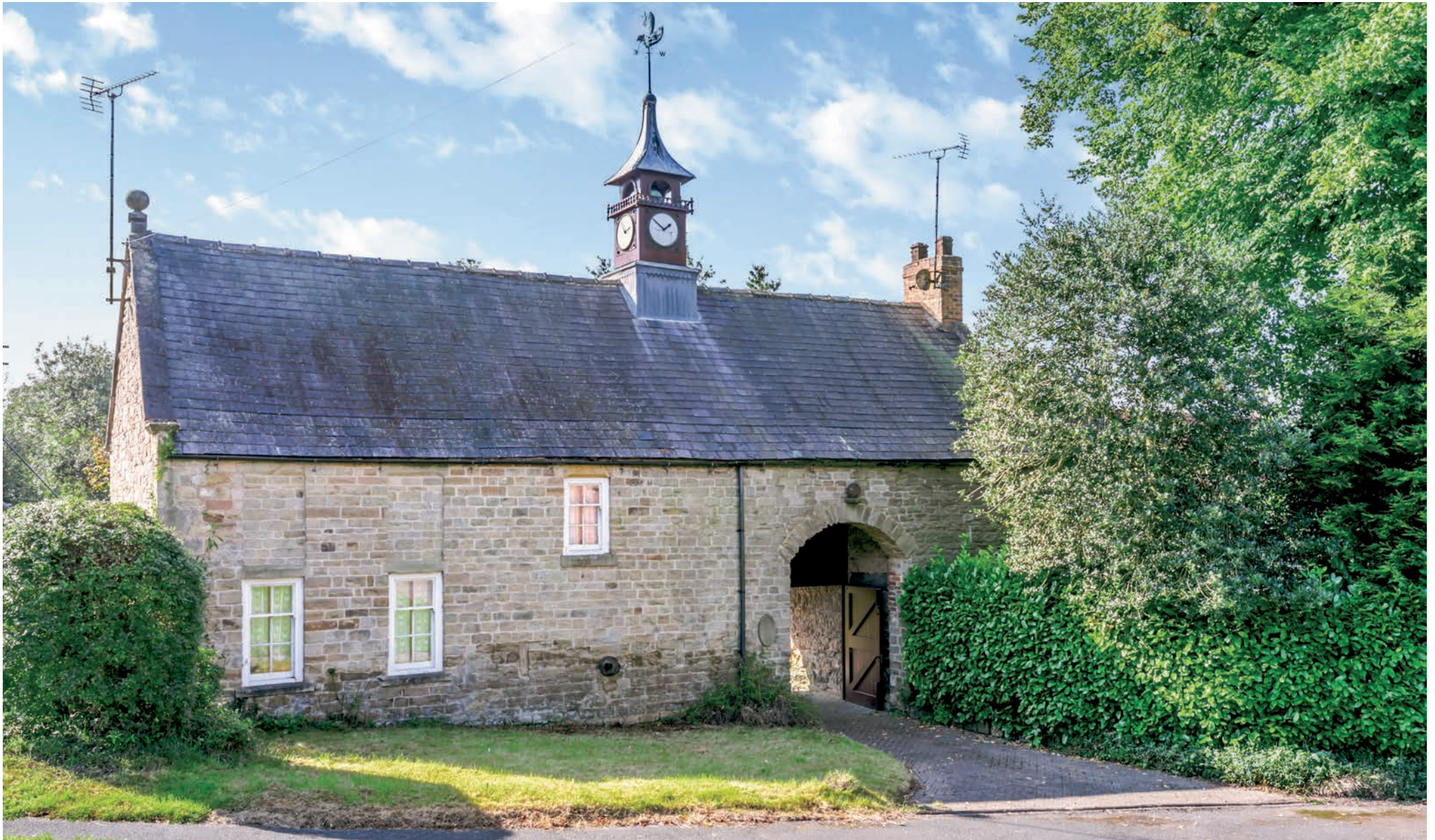
The Coach House Church Street | Barlborough | Chesterfield | Derbyshire | S43 4EP
