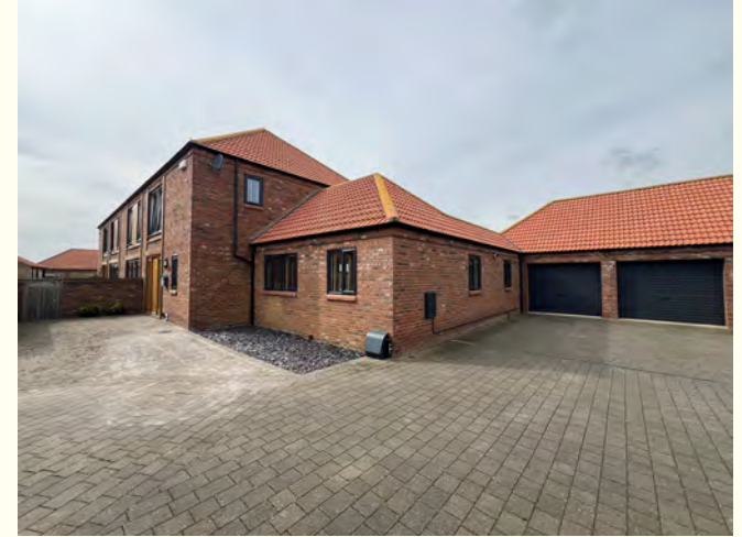
Driveway and Double Garage
